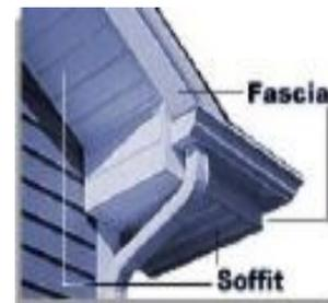
A finish member around the face of eaves and roof projections. Horizontal boards attached to rafter/truss ends at the eaves and along gables. Roof drain gutters are attached to the fascia.
